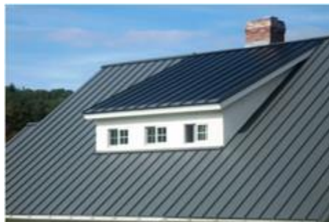
Figure 19-11: Building-Integrated Solar Energy System
