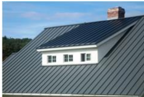
Figure 19-11: Building-Integrated Solar Energy System
